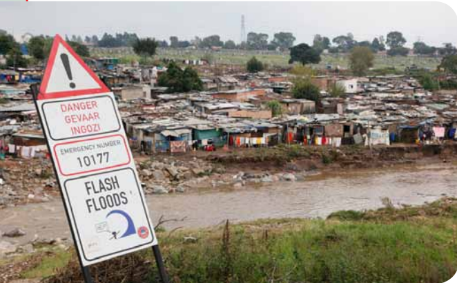
The scene of frequent disastrous floods
